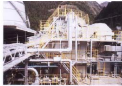
Wood Chip Burning Boiler
