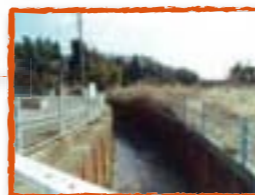
Left: Before improvement (location about 300m from right photo); Above: After removal of concrete banks and adjustment of river width to match natural terrain (Shinichi Yoshimura)
