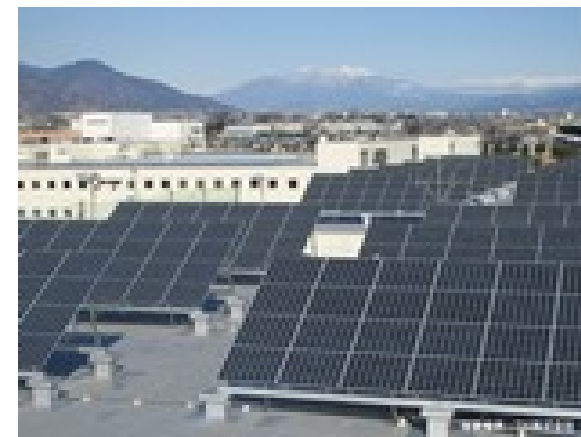
Large-scale solar panel installation on plant roof
