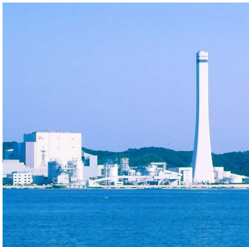
Tachibana Bay coal thermal power plant, Japan's largest
