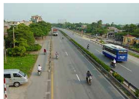
National Highway No. 5 in Hai Duong Province
