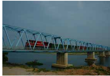
Thach Yuan Bridge on the Hanoi-HCMC line in Phu Yen Province
