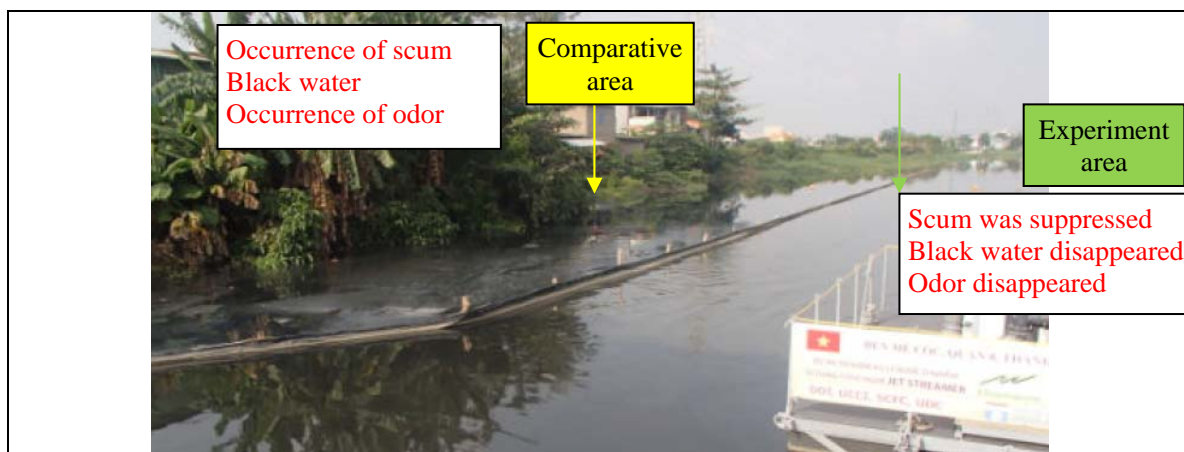
Fig3 Effect by installation of water flow generator “Jet Streamer”
