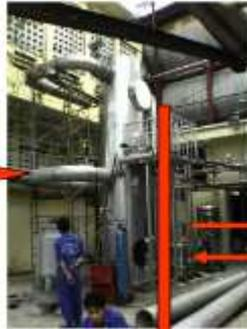
Scrubber: cleans the waste steam and generates hot water for pre-heating the wort for the following batch
