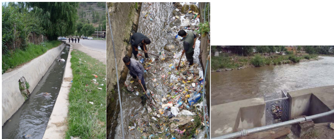
Photo6: near Veg. market ditch Center: Rubbish sweeper in ditch at city center Right: Renewed ditch outlet to Wang chhu
