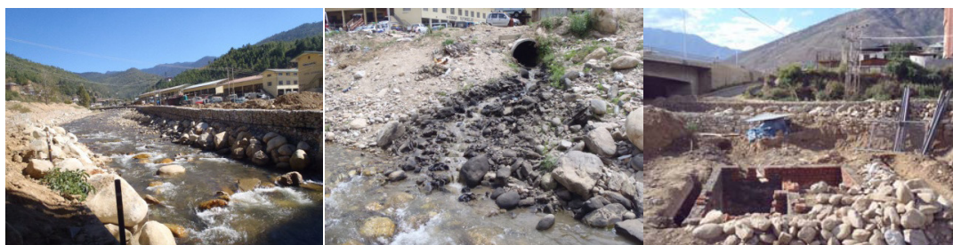
Photo7: Ola rongchhu Center: Oil flow from workshop Right: Construction of oil-catcher
