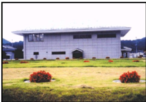
Nantan city treatment plant
