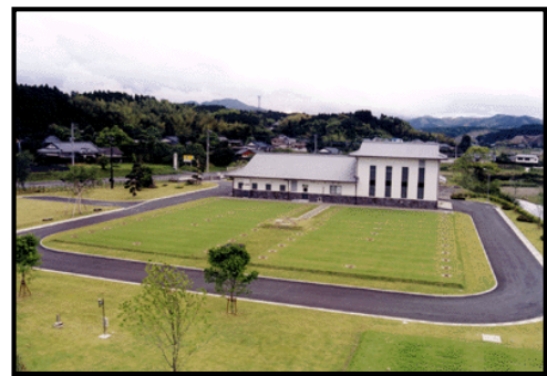
South kyusyu city treatment plant
