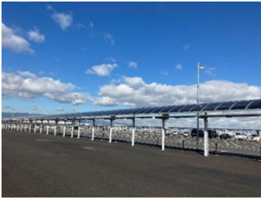
Perovskite solar cells installed at EXPO, Osaka-Kansai Transportation Terminal (Photo: Ministry of Economy, Trade and Industry)
