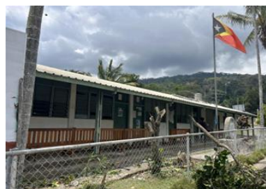
A health center in the project area.
