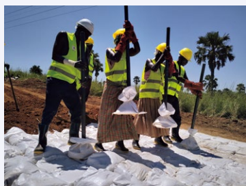
Road repair training using Do-nou technology (Photo: CORE)
