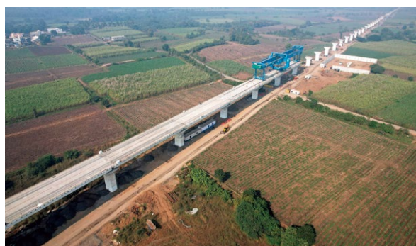
Full span casting (a method for construction of viaducts) as part of the “Project for the Construction of Mumbai-Ahmedabad High Speed Rail” in India (Photo: National High Speed Rail Corporation Limited (NHSRCL))
