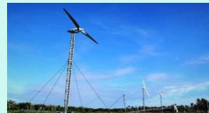
Development of tiltable wind turbines in Tonga (Photo provided by: JICA)
