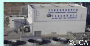
Navoi Thermal Power Plant (Uzbekistan)
