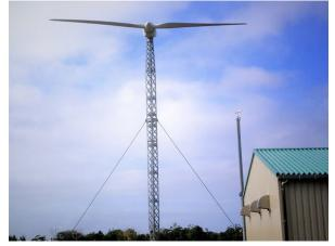
Tiltable wind turbine set up in Tonga through the Project for Installation of Wind Power Generation System (Photo: JICA)
