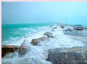
The causeway before reconstruction, affected by waves at high tide (Photo: JICA)
