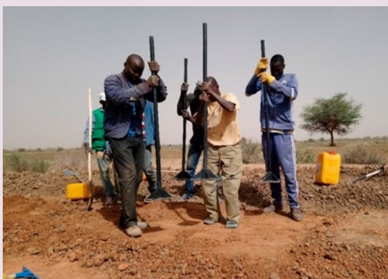
Conducting waterway compaction work as part of a farmer-participatory construction work in the department of Podor in January 2018 under the guidance of SAED (National Company of Development and Exploitation of Land in the Delta of Senegal River, and Faleme Valleys) extension officers who had received the leader's training on maintenance and management under PAPRIZ2 (Photo: JICA)
