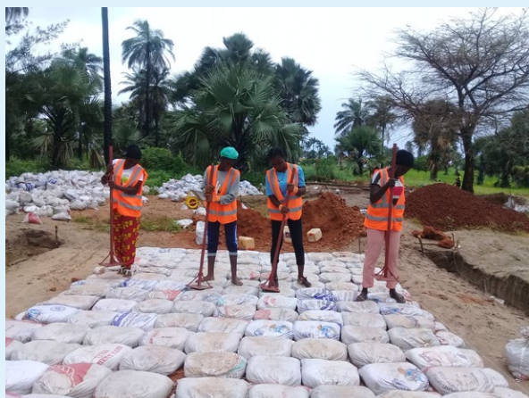
Women compacting Do-nou bags to create the road base (Photo: CORE)
