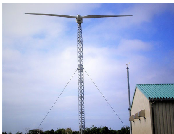
Tiltable wind turbine set up in Tonga through the Project for Installation of Wind Power Generation System (Photo: JICA)
