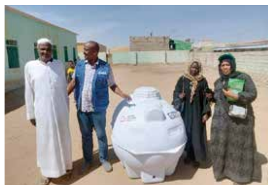
Water tanks installed at an evacuation shelter, enabling regular water supply assistance
