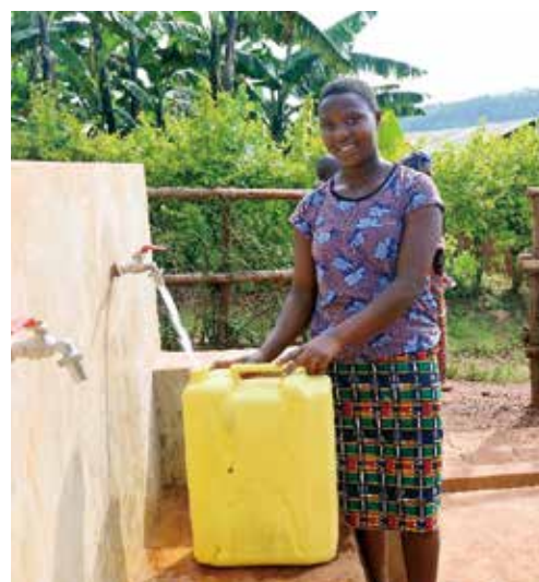
A water point constructed under the project and maintained by the water user committee in the village
