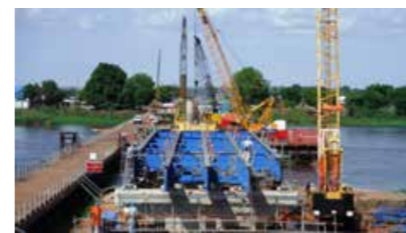
Bridge under construction
