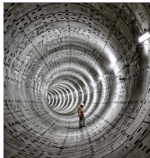
Breaking Ground A Narrative on the Making of Delhi Metro
