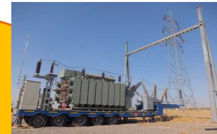
Mobile Substation
