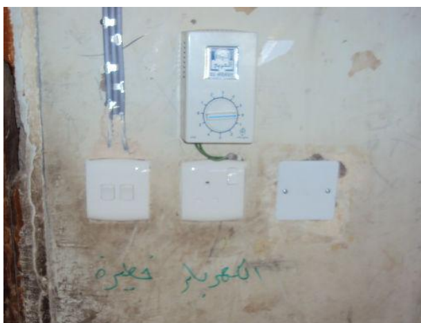
校内電気設備修復後 (Al-Hayat school)
