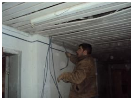
電気設備修復 Al-Hayat school (2011.12 & 2012.3)
