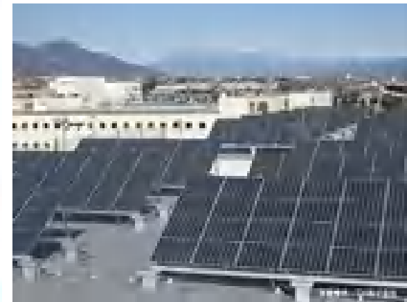
Large-scale solar panel installation on plant roof
