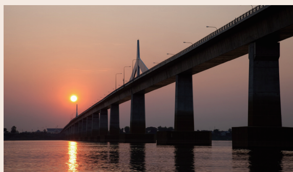
Laos: Second Mekong International Bridge over the East-West Economic Corridor (Photo by Shinichi Kuno / JICA)
