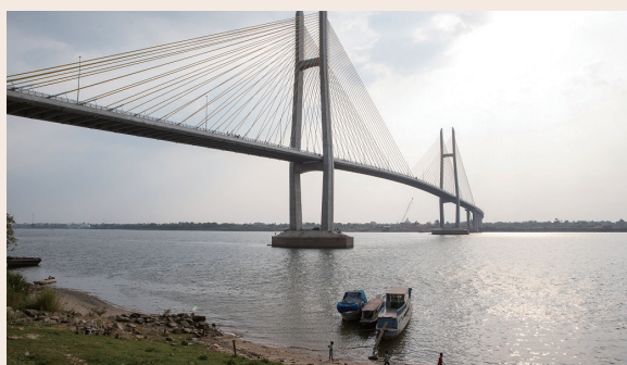
Cambodia: Tsubasa Bridge over the Southern Economic Corridor (Photo by Shinichi Kuno / JICA)
