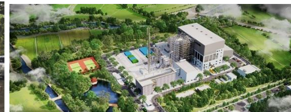
Waste-to-Energy Plant in Vietnam
