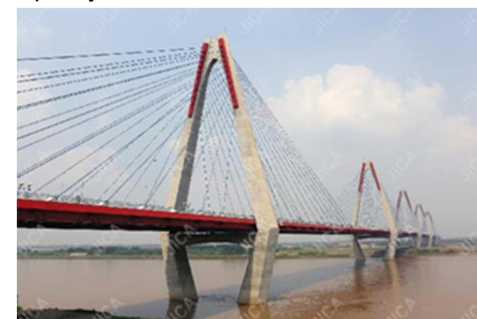
Vietnam “Nhat Tan Bridge (Vietnam-Japan Friendship Bridge) Construction Project”
