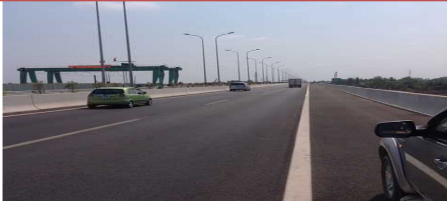
North-South Highway in Viet Nam (Provided by JICA)
