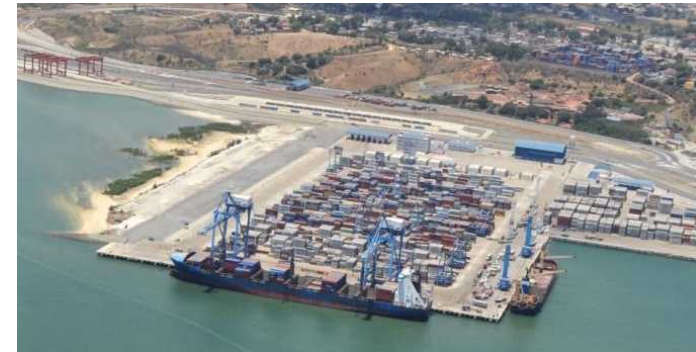
New container terminal at Mombasa Port in Kenya (Provided by TOYO CONSTRUCTION CO., LTD)
