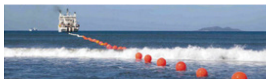
Laying optical submarine cable in the South Atlantic (Courtesy of NEC)
