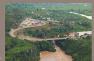
Rusumo Bridge 1 (Photo by JICA)
