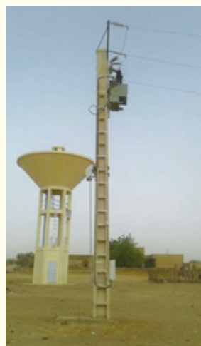
Water tower and power pole in Senegal
