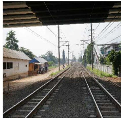
Ground, Double Track, Electrified
