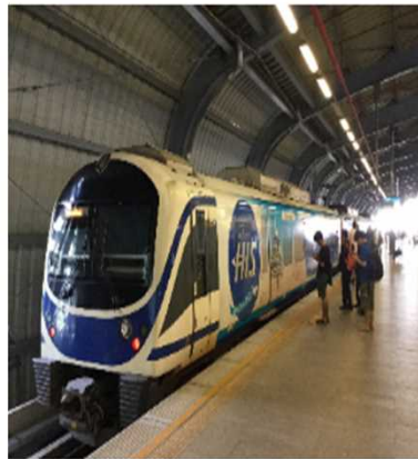
Elevated, Double Track, Electrified
