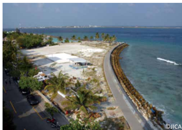
Seawalls built around the Male Island
