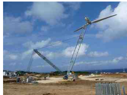
Wind turbine tiltable system
