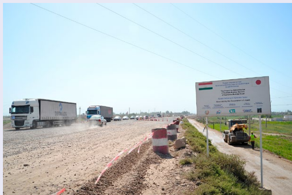
The road during construction. The road was unpaved and had no sidewalks. (Photo: JICA)
