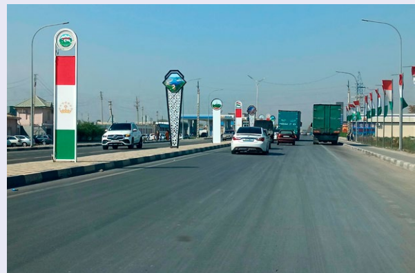
The road after completion. Sidewalks, fences, central medians, and street lights have been installed, ensuring traffic safety. (Photo: JICA)
