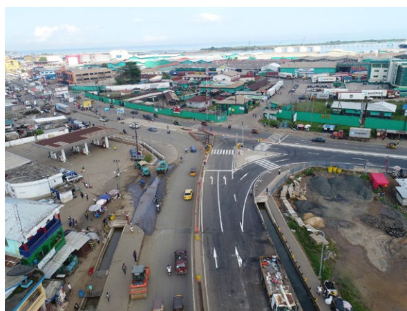
The “Japan Freeway,” a highway in Liberia that Japan has been engaged in constructing and rehabilitating since 2013 (Photo: JICA)
