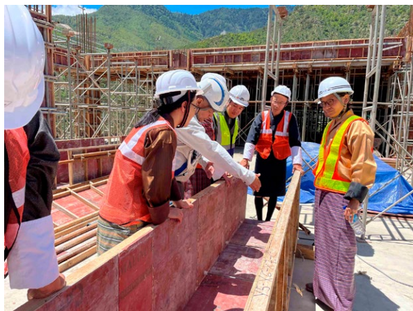
Strengthening the capacity of engineers in the construction sector as part of the technical cooperation, “Project for the Establishment of Human Resources Development System in Construction Sector” in Bhutan (Photo: Oriental Consultants Global Co., Ltd.)
