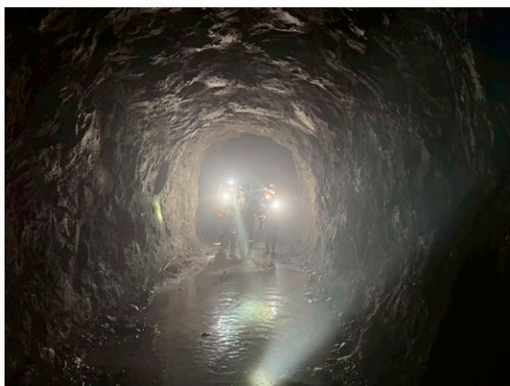
Survey inside the Sekisovskoye gold mine (Photo: Hokkaido University)
