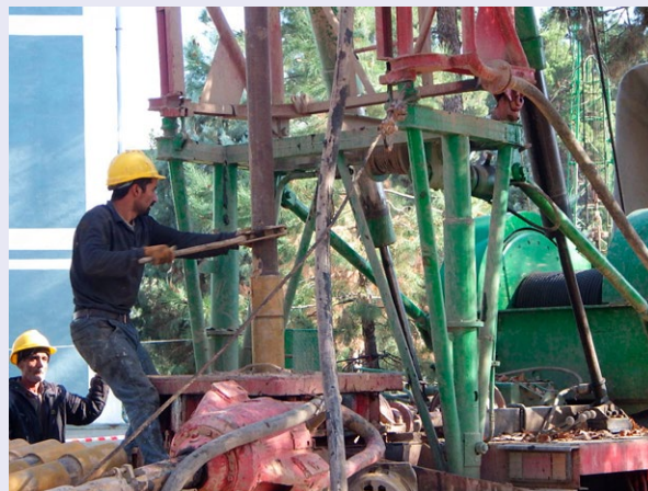
Well drilling work at the second demonstration site (Machiton) (Photo: Japan Groundwater Development Co., Ltd.)
