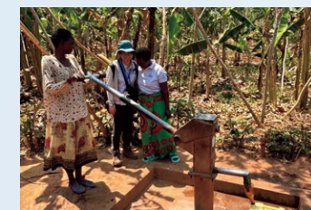
The author (second from left) celebrating with the village chief after the successful completion of well repairs
