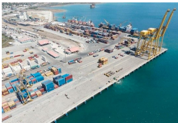
The Nacala Port in Mozambique, where Japan is advancing port development and functional enhancement (Photo: Penta-Ocean Construction Co., Ltd. & Toa Cooperation Joint Venture)
