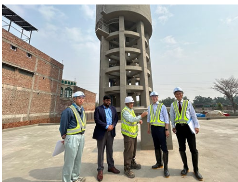
Water distribution facilities installed under the "Project for Improvement of Water Treatment Plant and Water Distribution System in Faisalabad," the city which has the third-largest population in Pakistan
