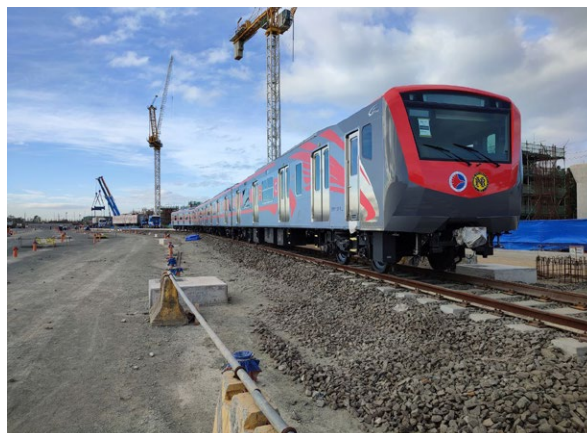
The yen loan project “North-South Commuter Railway Project (Malolos–Tutuban)” in the Philippines is contributing to the alleviation of serious traffic congestion in Metro Manila. (Photo: JICA)
