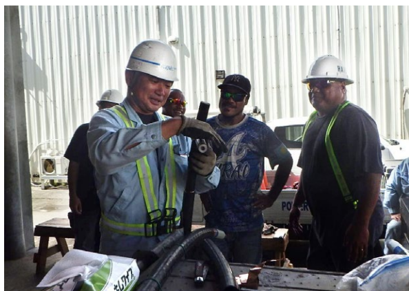
A Japanese company engineer instructing staff of the Palau Public Utilities Corporation (PPUC) on terminal processing for underground cables, as part of the grant project “The Project for the Development of Power Transmission Network” for Palau (Photo: TOENEC Corporation International Division)
