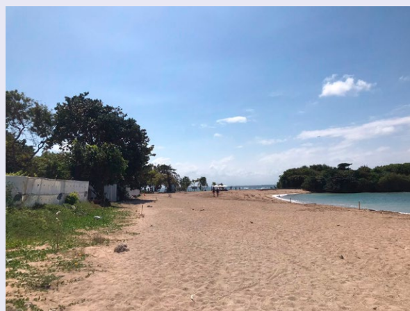
Nusa Dua Beach after the project, with the seawall and sandy beach restored (Photo: Nippon Koei Co., Ltd.)
