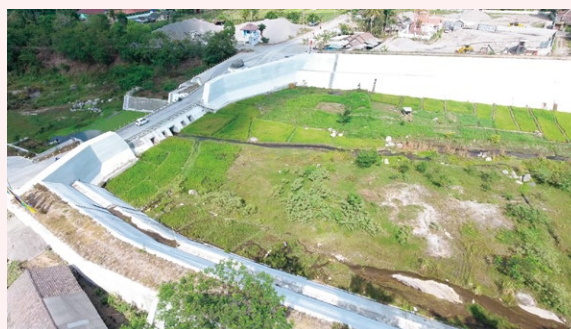
A sabo dam that is used as a bridge during normal times (Photo: Yachiyo Engineering Co., Ltd.)
