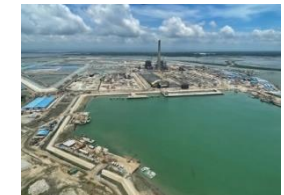
Matarbari deep-water port (Bangladesh)
