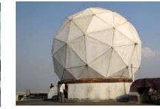
Bangladesh: Improvement of the meteorological radar system
