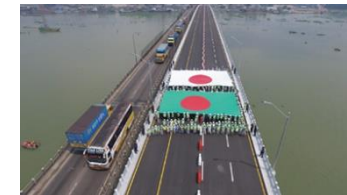
Meghna 2nd Bridge (Bangladesh) (Photo credit: OBAYASHI Corporation, Shimizu Corporation, JFE Engineering Corporation, and IHI Infrastructure Systems Consortium)
