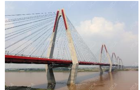
Vietnam “Nhat Tan Bridge (Vietnam-Japan Friendship Bridge) Construction Project”
