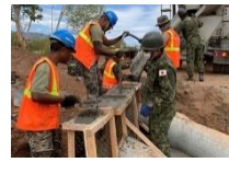
Timor-Leste: Civil engineering
