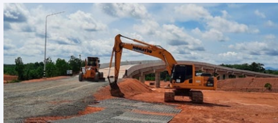
Road construction using high-precision positioning data and ICT construction machinery (Photo: JICA)
