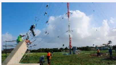
Construction of an antenna for an AM radio broadcasting system that enables information communication to the Niua Islands, approximately 600 km from the capital (Photo: JICA)
