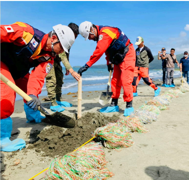
Japan Disaster Response Relief Expert Team installation of oil snares for heavy oil absorption in Mindoro © JICA
