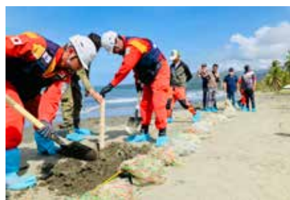
Japan Disaster Response Relief Expert Team installation of oil snares for heavy oil absorption in Mindoro © JICA
