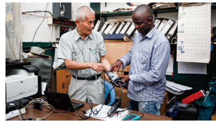
JICA Expert Teaching Local Technician How to Use Instruments at a Transformer Station in Sierra Leone (Photo: Iizuka Akio/JICA)
