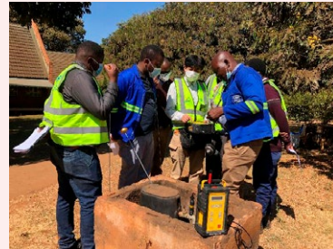
Mr. Sekimoto providing guidance on technology for detecting underground water leakages (Photo: JICA)
