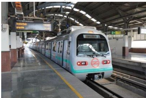
India “Delhi Mass Rapid Transport System Project”
