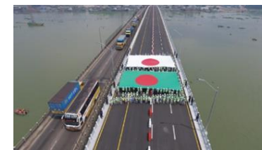
Meghna 2nd Bridge (Bangladesh) (Photo credit: OBAYASHI Corporation, Shimizu Corporation, JFE Engineering Corporation, and IHI Infrastructure Systems Consortium)
