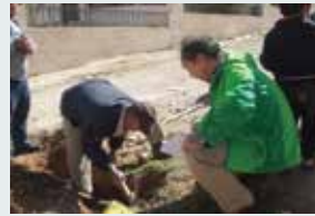
Project for formulating water supply plan for the host communities of Syrian refugees (2013-2016)
