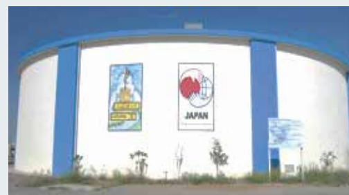
Improvement of the Water Supply System for the Zarqa District (FY 2002-2003, 2006-2008: 4,092 million yen)
