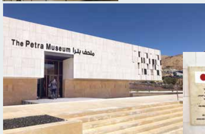
Construction of Petra Museum (Cultural Grant Assistance) (FY2013-2014: 784 million yen)
