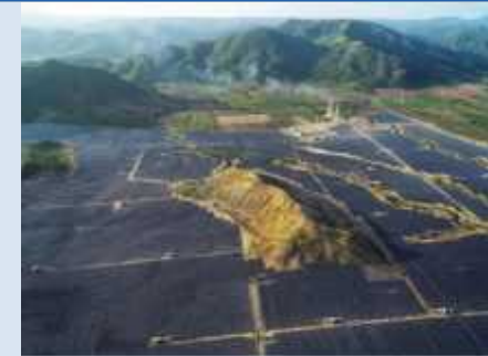
Viet Nam: Solar Power Generation Project
