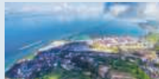
Sihanouville Port in Cambodia (Photo: JICA)
