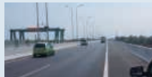
North-South Highway in Viet Nam (Photo: JICA)
